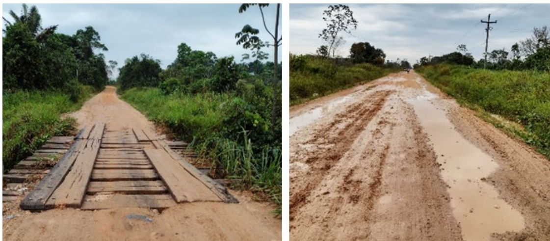
Fig. 4. Access roads - Campo Verde
